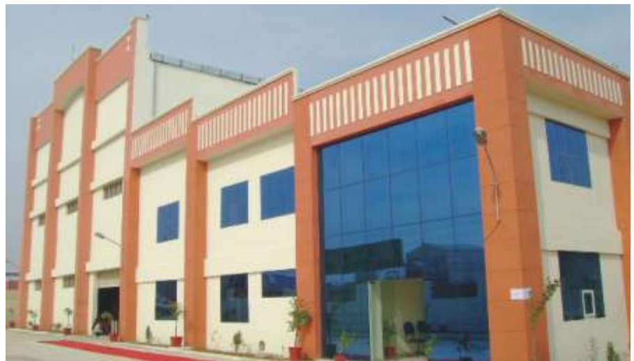
LATICRETE® Plant, Sotanala, Rajasthan
