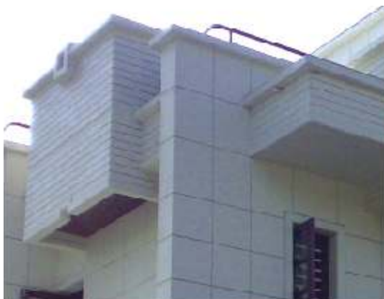
Vitrified Tiles Installed on an External Facade
